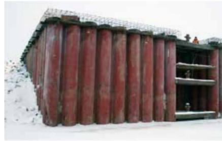
O-Pile systems are a rapidly expanding construction method that utilize pipes to form extremely strong foundations, barriers and retaining walls in a cost-effective way.
